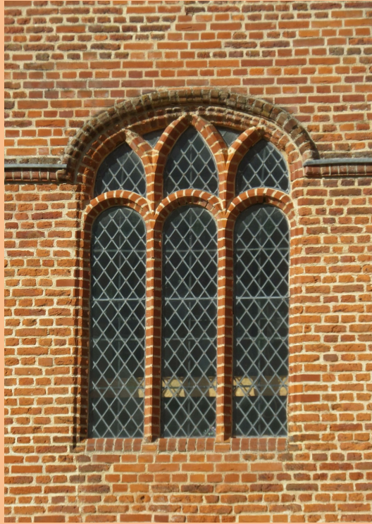
St Mary's 1629 bell-tower window, with local red building- and rubber-bricks
